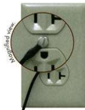
Figure 10, attachment of ring terminal to ground
